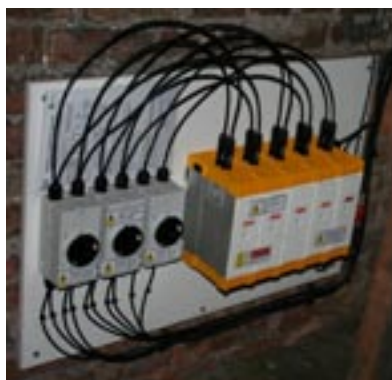
Five inverters and the meter
